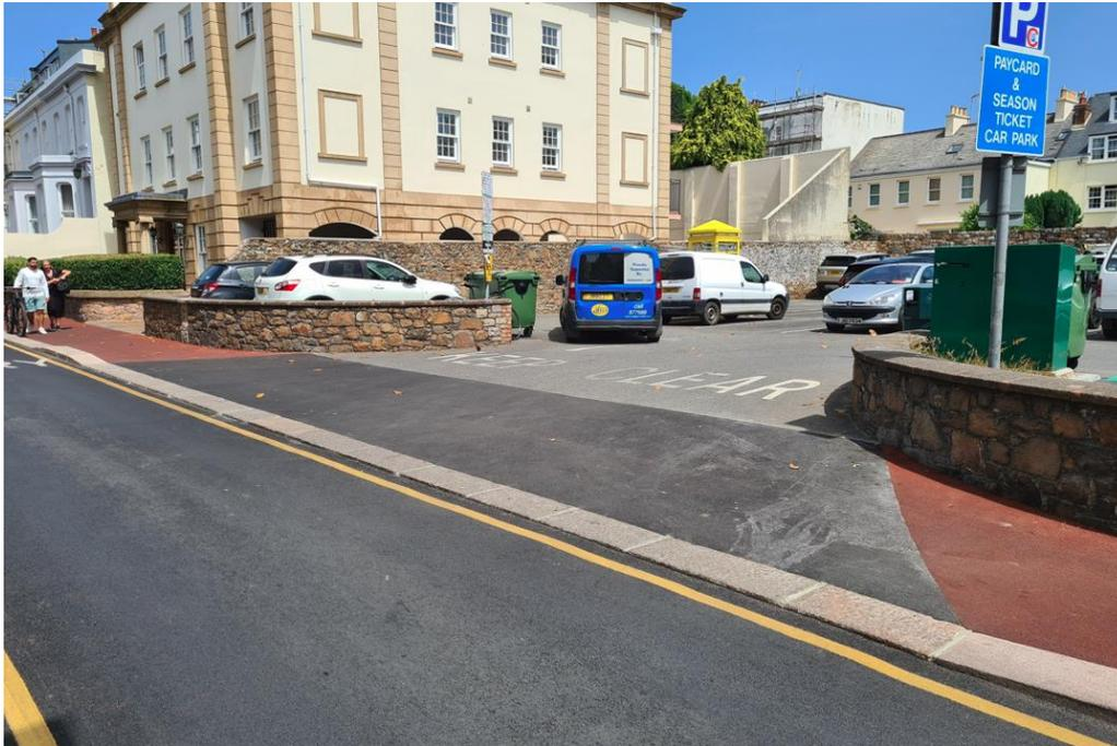
The Parish Roads Committee does not support the approach as illustrated in the photo above, as this gives the wrong message that motorists have priority across the footpath due to the red asphalt being stopped at either side of the vehicle entrance.
